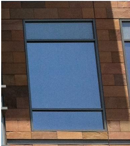
Figure 4: Typical Window at RFCS
